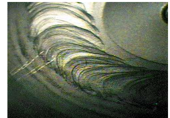
View through borescope
