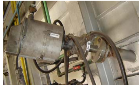
Furnace Camera with F31 Flange Mount
