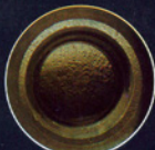
Photograph of closed, seated valve after cleaning.
