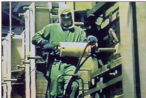
Fig. 1 Wearing fire-retardant gear, a technician inserts the periscope of the CCTV system into the regenerator chamber of a glass furnace to view checker packs used to regenerate heat during manufacture of glass.
